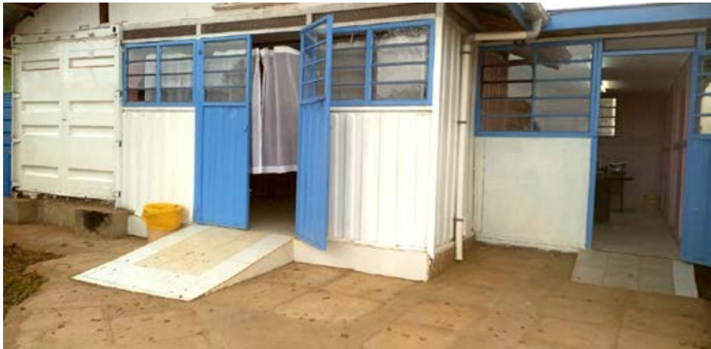
Structure of Kajiado GBVRC located at Kajiado County Referral Hospital. File
